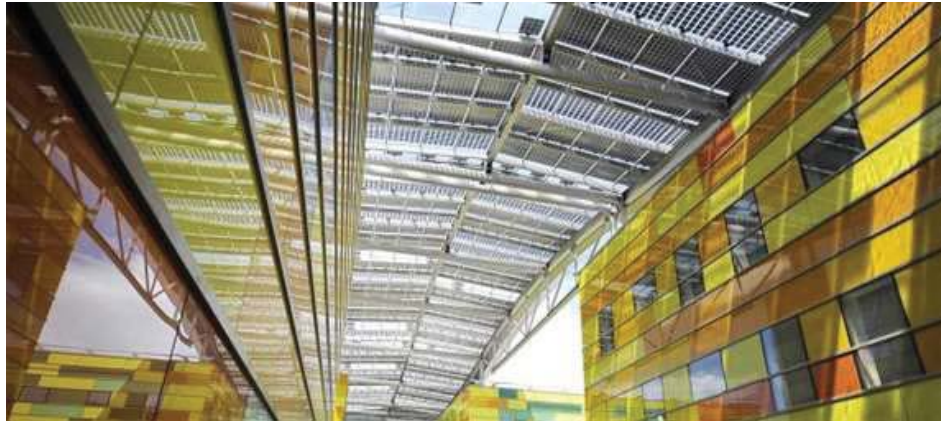
Figure 4.1 - Example of BIPV system applied to the roof (spaced PV cells allowing the passage of natural light) - Gare de Perpignan, France (Révolution Énergétique, 2022).
